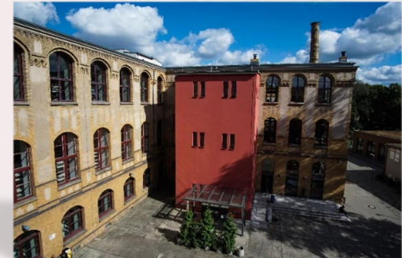
Campus Nord branch library entrance area
